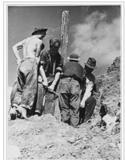
Young men of the CCC at work, c. 1933, Virginia.
